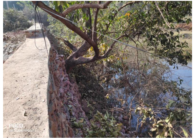
Photo showing guard wall to arrest silt going to nalla
