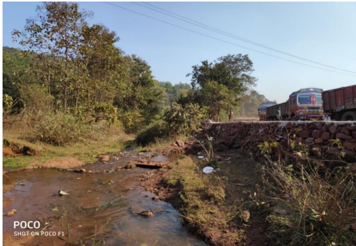
Photo showing guard wall to arrest silt going to nalla
