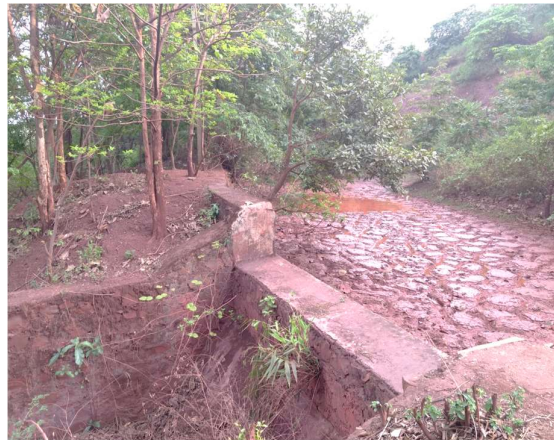
Pic 6- settling pond and check dam.
