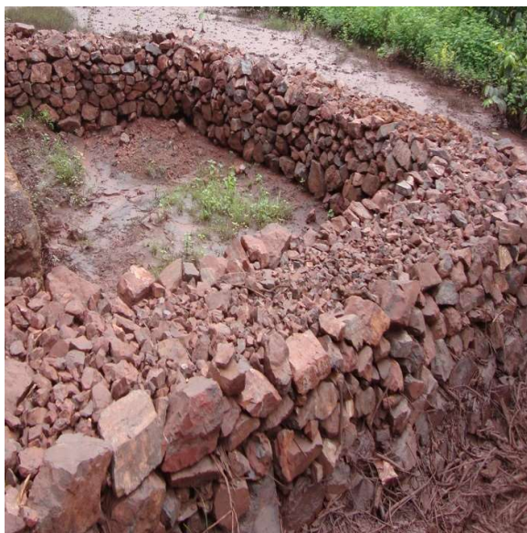
Pic 7- Check weirs near bank of Nallah
