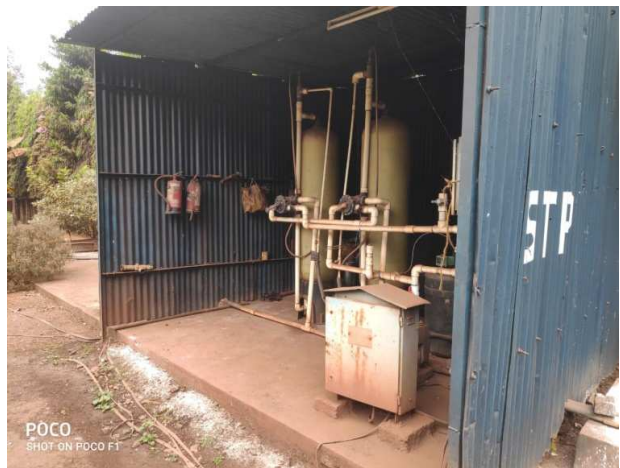
Photo#07: Sewage Treatment plant (Ultra filtration unit) at Staff campus
