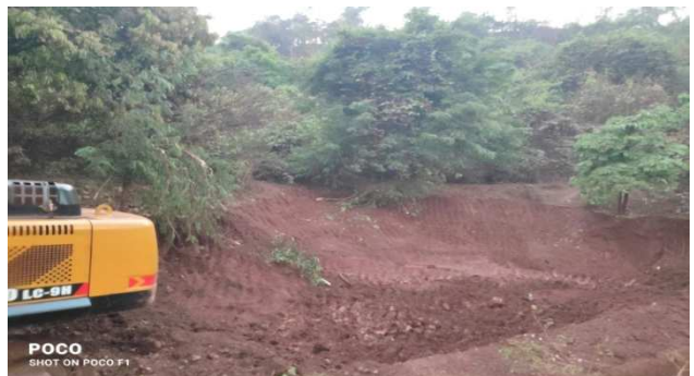
Photo#04: Guard wall, garland drain, settling pond and its de-silting
